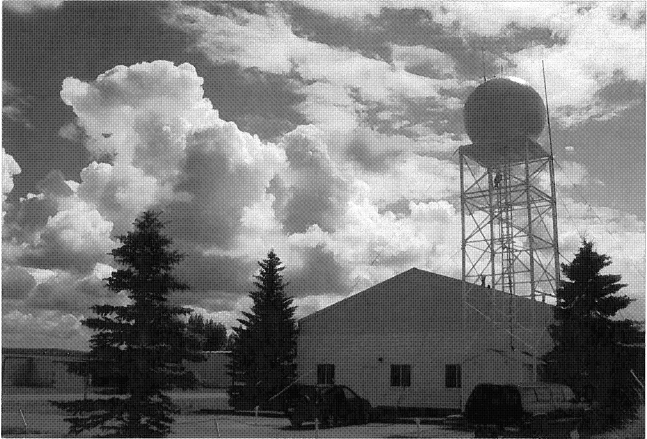
Fig. 21. The project Operations Centre at the Olds-Didsbury Airport. WMI photograph by Bradley Waller.
