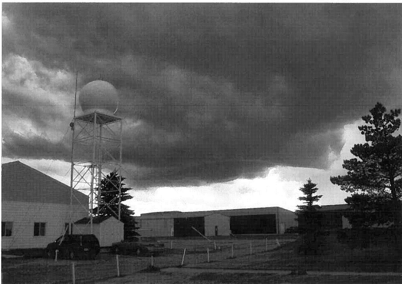
Fig. 14. The WMI project Operations Centre is located at the Olds-Didsbury Airport, about 70 km (44 miles) north of the Calgary Airport, roughly halfway between the project's most important cities: Calgary and Red Deer. The radar antenna is housed within the dome, and the transmitter and receiver in the shed at the tower base. Operations are conducted from within the meteorological office housed within the adjacent hangar. In this image from 7 June 2013 at 4:36 PM, the darkening, yet rain-free cloud base overhead signals the organization of updrafts ferrying moisture into the developing storm above. WMI photograph by Bradley Waller.
